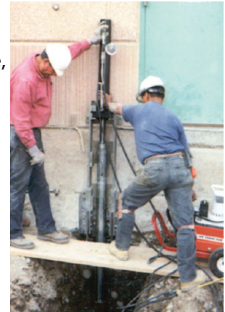
Installation by smooth hydraulic pressure extends pier to reach competent end-bearing soil stratum.
